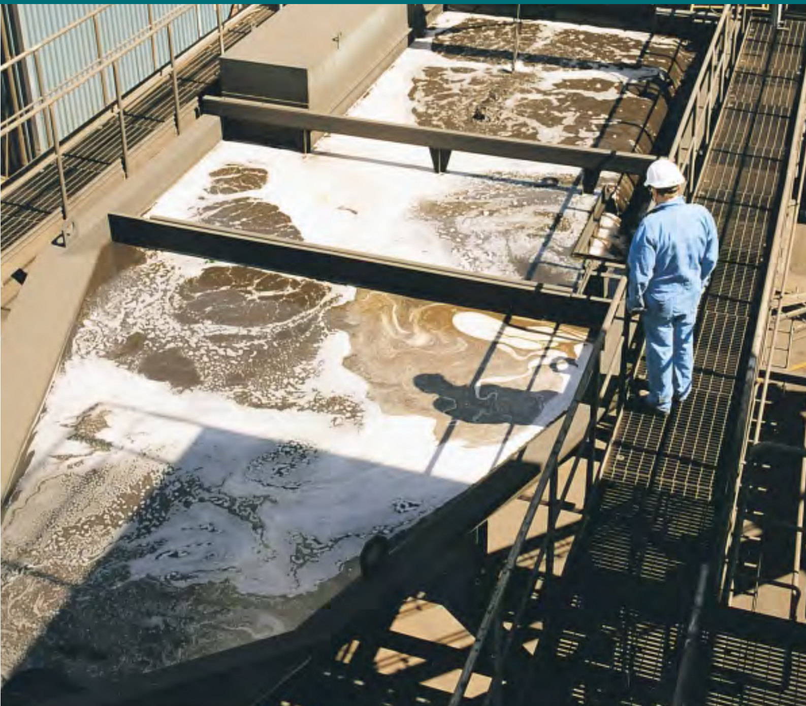
Feed distribution in a SD60-200.
