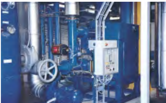
Metso HGMF for control of magnetic concentration in a district heat flow of 10.000 m 3 /h (44000 USGPM)
