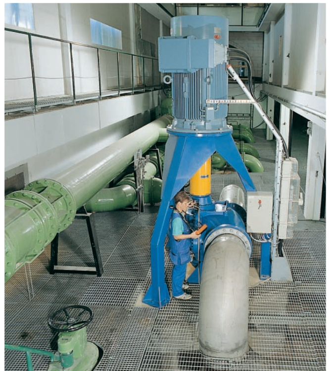
Vertical shaft pumps are often installed in water works.
